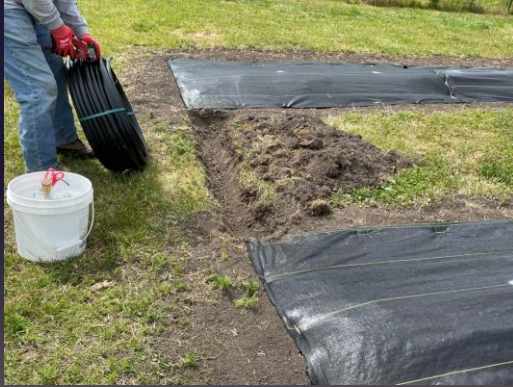
Installing main poly tubing
