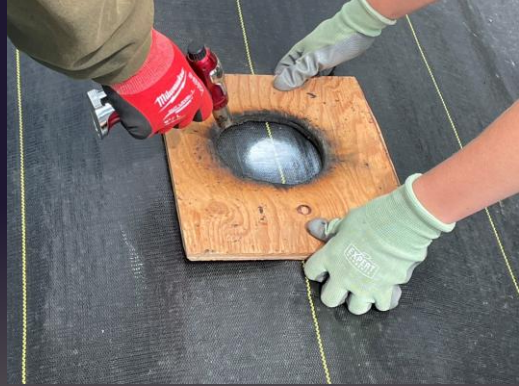
Burning hole with template
